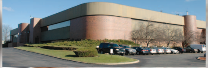
Narda Microwave Headquarters, Hauppauge, New York
